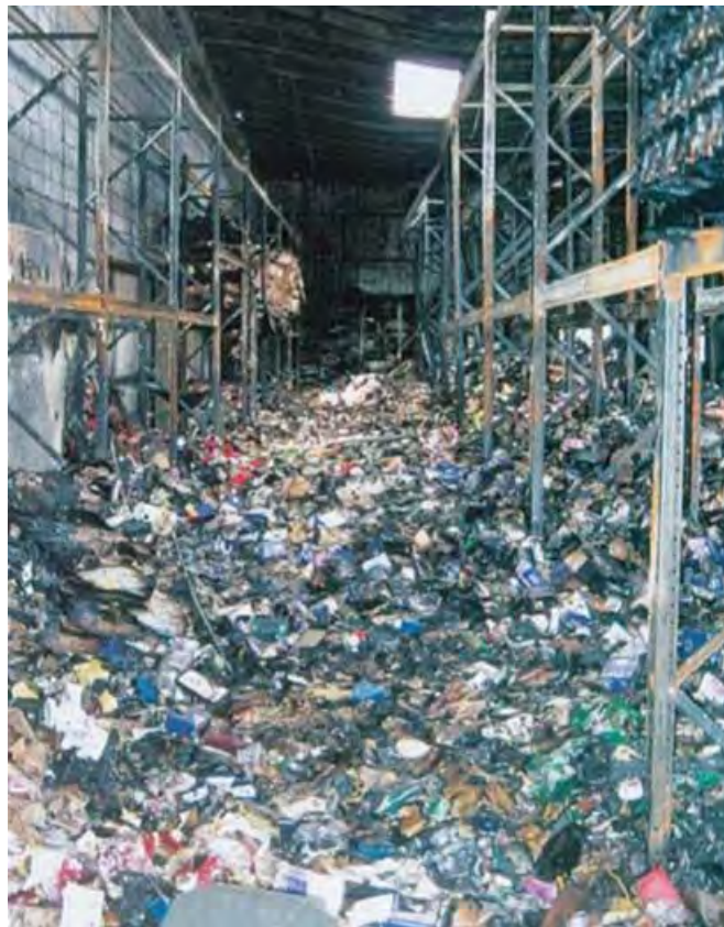
Fig 5.2.49: Results of a Fire in a Perfume Warehouse
