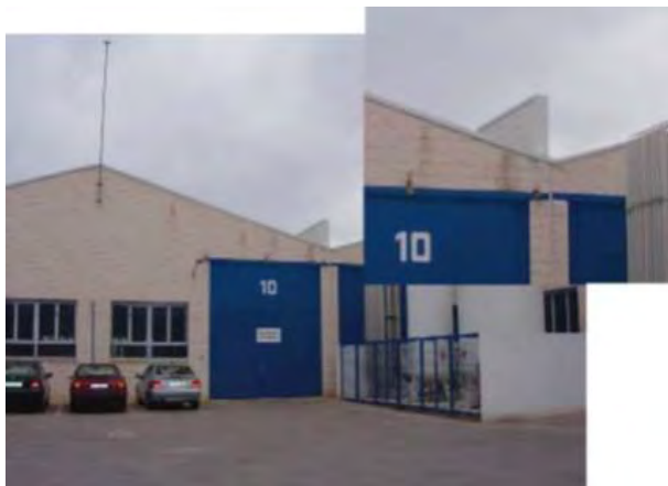
Fig 5.2.67: A dividing wall separating two buildings
