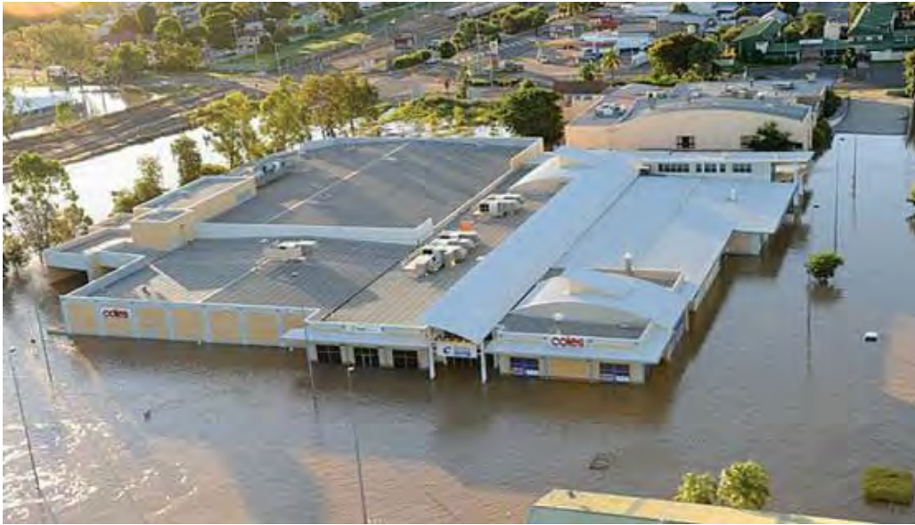
Fig 5.2.75: Flood water surrounding a warehouse
