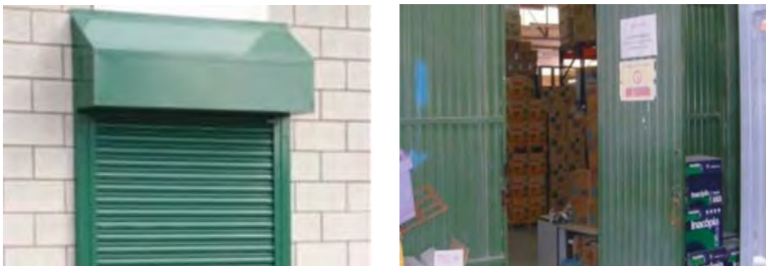
Fig 5.2.78: Lockable metal shutter warehouse door
